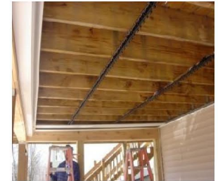
Install Side Cap & Flashing.
