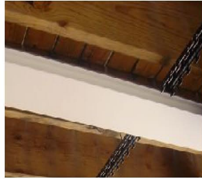
Temporarily set a panel to position G-Channel & Gutter
