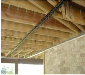
Temporarily set the Carrier
