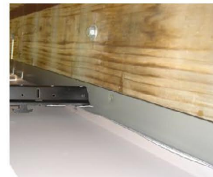
Fasten with single screw
