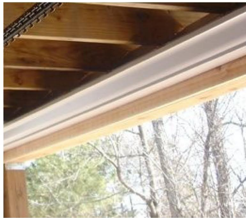
Install Gutter
