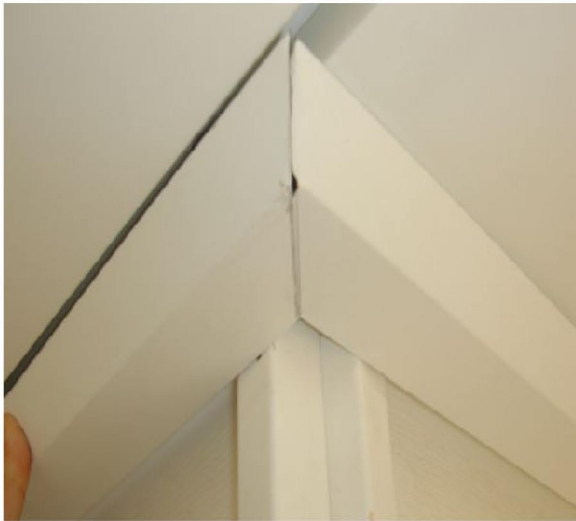
Outside miter of G-Channel
